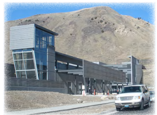
New transit vehicle maintenance facility (phase 1 complete)
