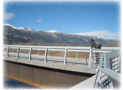
New Snake River bridge, part of the pathway network parallel to WY-22, opened in fall 2014
